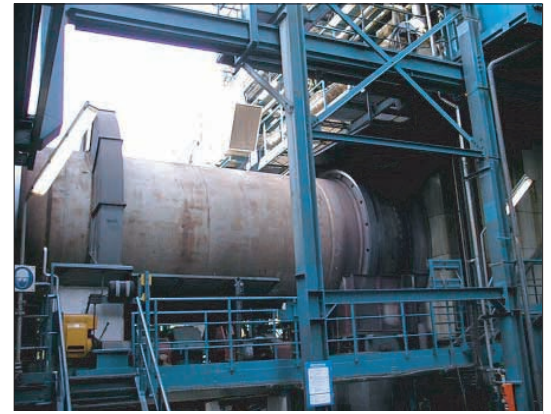
Figure 5a. View at the outer shell of KILN B.
